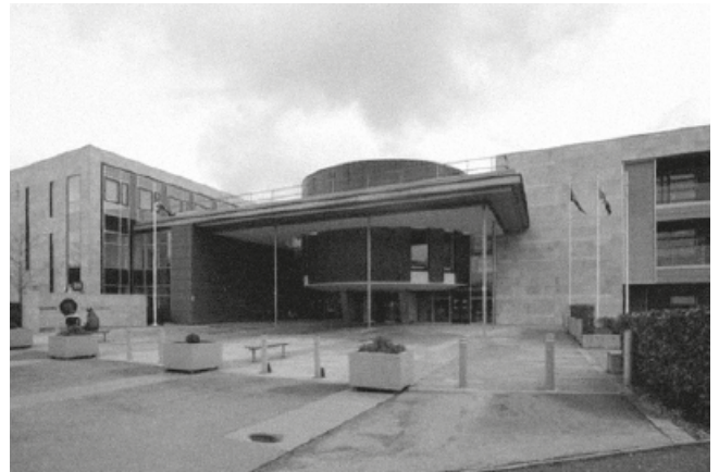
Livingston Civic Centre. This multi-agency site is perhaps the best example of co-location of statutory services in the UK and was the delivery site for day four of the programme.
